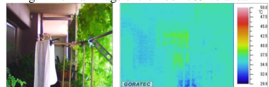
Fig.3 Thermal Image of the Room502 Veranda
