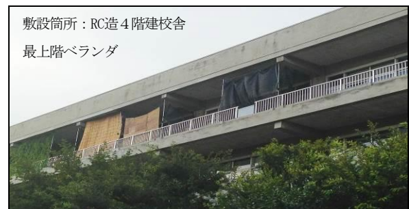
Photo 1 Balcony of the Nihon University
