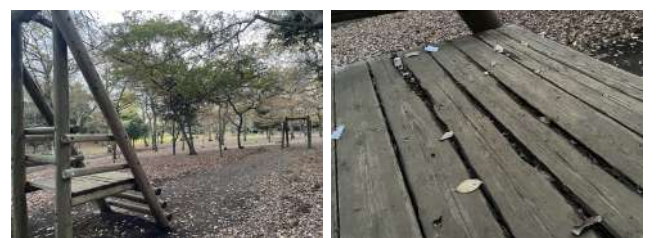
a) Entire playground equipment b) Floor surface used as a test piece Picture 1. Removed Wooden Ropeway
