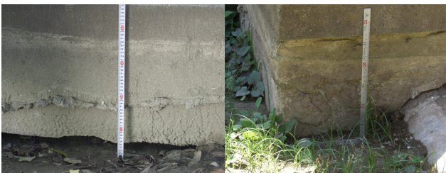
Fig.2 Measuring of settlement
