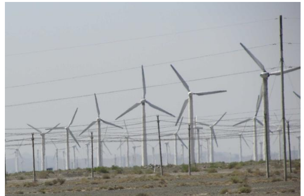
Photo1. Wind power generation facility in Torfan.
