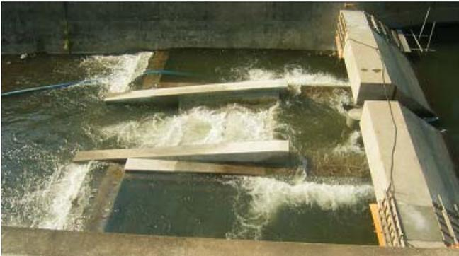
Photo 1 Fish facility installed in flood control weir
