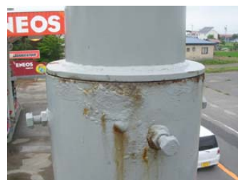
Figure 1. Example of corroded structure
