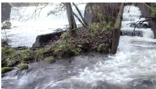
Photo 1 Flow conditions of fishway and check dam (before improvement) located in Shunkarikotan river
