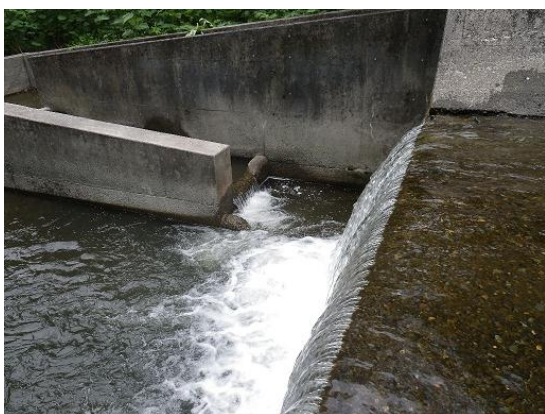
Photo 2 Interaction between the downstream end of fishway and aerated plunging flow region (check dam located in Monomanai river)
