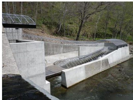
Photo 6 Flow condition immediately downstream of Check dam in Shunkarikotan river
