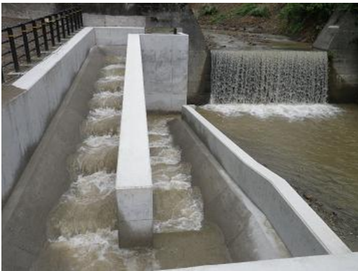
Photo 5 Flow condition immediately downstream of Sabo dam in Aikawa river
