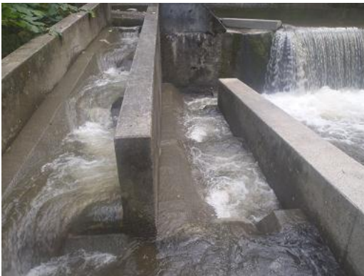
Photo 4 Flow condition immediately downstream of Check dam in Monomanai river
