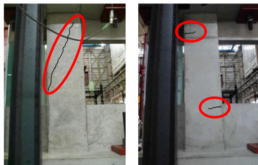
Photo.1 typical cracking patterns at R=+5/1000rad
