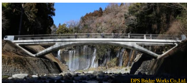
Photo 1. The Subject Bridge
