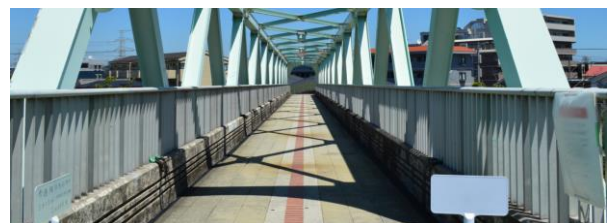
Photo 2. The Subject Truss Bridge
