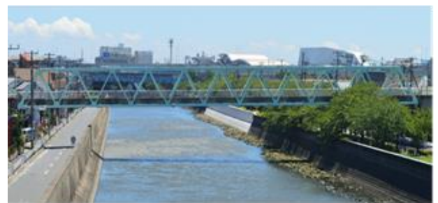
Photo 1. The Subject Truss Bridge
