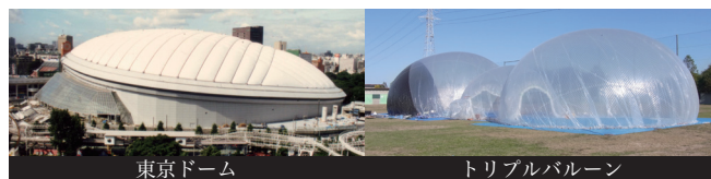
Fig.1 Examples of Building
