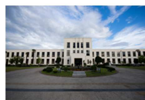
Figure3. Old school building
