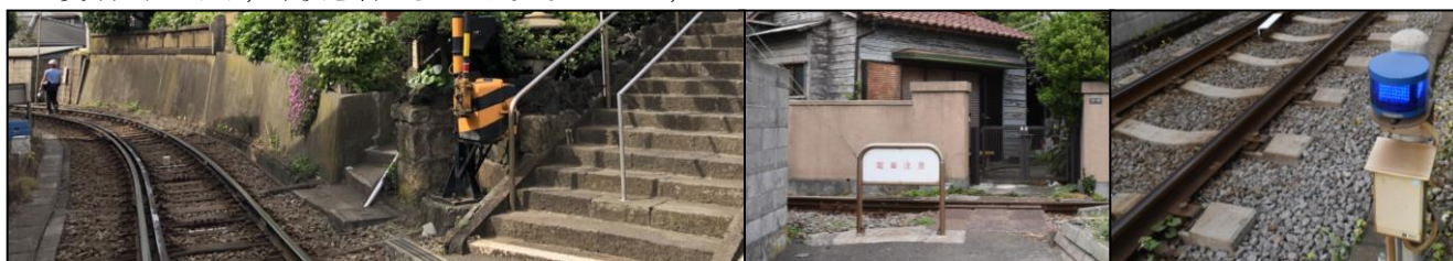
Photo1 One case study of the railway front entrance housing (線路側玄関住宅一例) (Photo by authors) Photo2 Simple pass and Attention sign (簡易的通路及び注意書き) (Photo by authors) Photo3 Warning lamp (警告ランプ) (Photo by authors)
