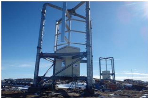
Figure1. 20 kW Windmill of Syowa Station [1]
