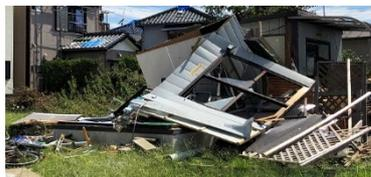
Fig.11 Collapse of prefabrication hut
