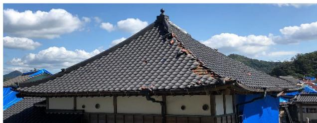
Fig.6 Fall of corner roof tile
