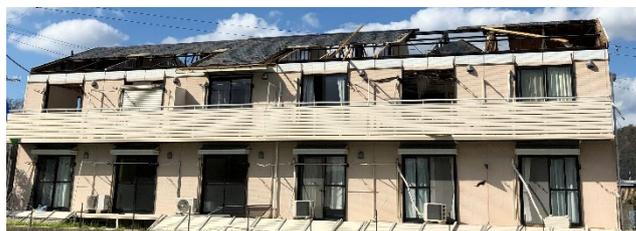
Fig.8 Destroyed Apartment house roof
