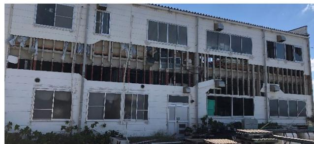
Fig.4 Damaged outer wall
