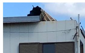
Fig.10 Metal roof peeling
