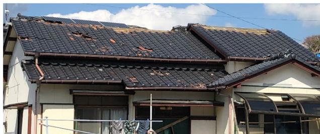
Fig.5 Fall of roof tile
