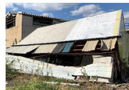
Fig.12 Collapse of warehouse
