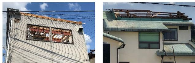
Fig.7 Destroyed wooden building roof
