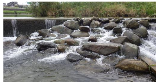
Figure 2. Fish passage with natural stacked boulders in Murasaki River
