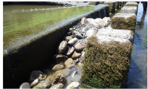
Figure 1. Fish passage with natural stacked boulders in Kuji River
