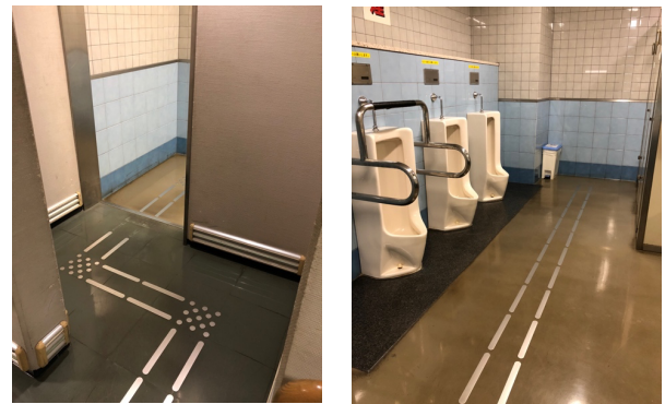
Figure 1. Installation status of Braille plates in the toilet
