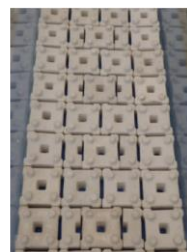
Figure 1. The installation of rugged blocks
