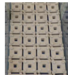
Figure 1. The installation of rugged blocks
