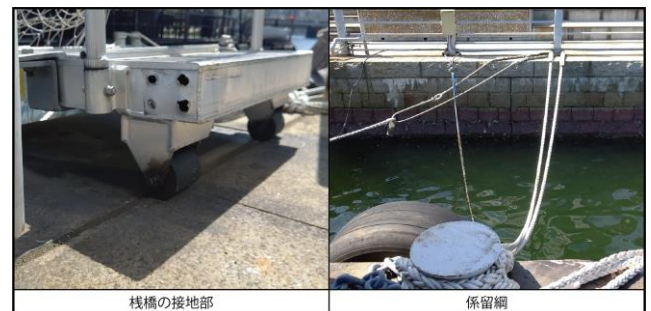
Photo 1. Pier grounding section and mooring rope
