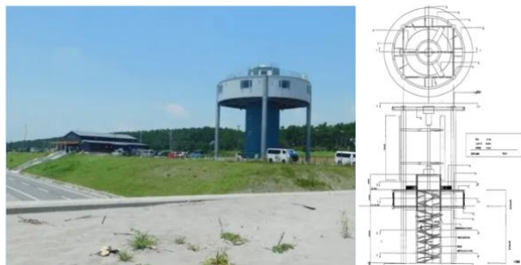
Figure4. Nagisa Exchange Center Tsunami Evacuation Tower
