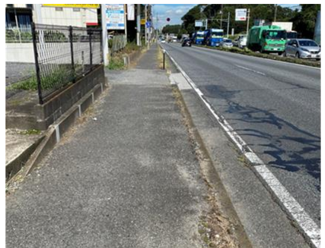
Figure 1. Picture of target sidewalk surface
