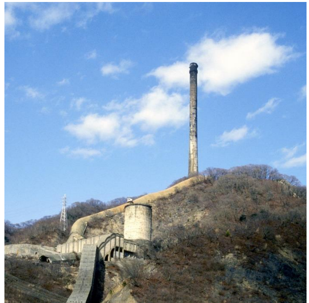
Figure 4. Large chimney at that time
