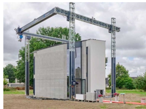
Figure 2. Example of 3D-print house in Belgium
