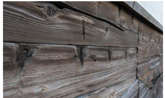
Photo.1 Nagahama City Boat Board Architecture
