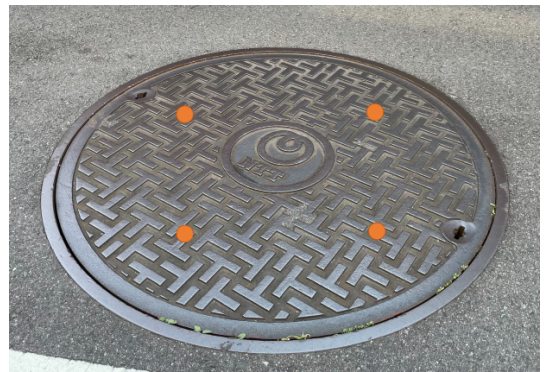
Figure 1. Example of measuring points with calipers
