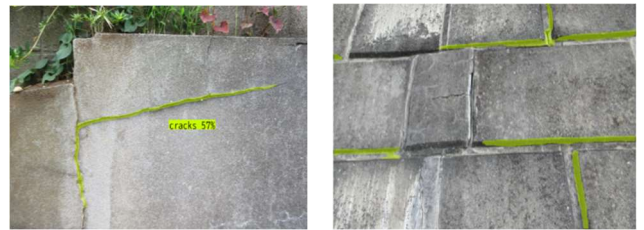
Concrete retaining wall
