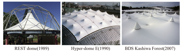
Figure 1 Typical Horn-Shaped Membrane Structure
