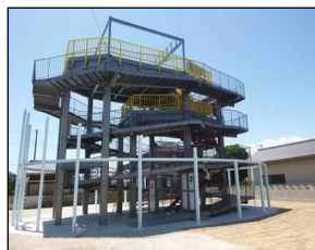
Fig.2 Tsunami evacuation tower
