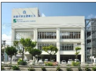
Fig.1 Tsunami evacuation building
