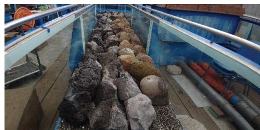
Photo 2 Installation of assembled boulders (left side Slag).
