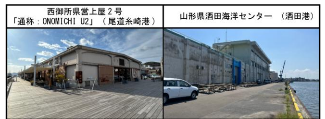
Photo.2 Facility of Minato Oasis
