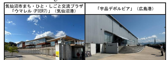
Photo.1 Facility of Minato Oasis
